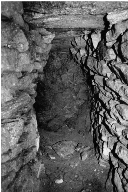
FIGURE 2. END OF SOUTERRAIN SHOWING CORBELLED CONSTRUCTION. PHOTO: M. PEARSON
