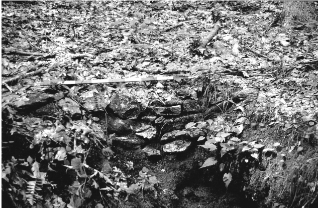
FIGURE 6. COURSES OF STONE COVERING CAPSTONES.
