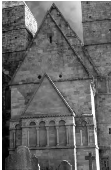
FIGURE 3. CORMAC'S CHAPEL ON THE ROCK OF CASHEL, IRELAND SHOWING FLUE OUTLETS ON THE EXTERIOR WALL. CARLSON
