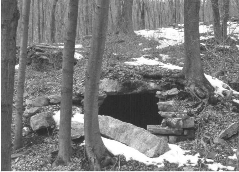
Figure 6. Photo of small chamber, showing fallen lintel across its entrance, in need of repair. The arc of long stones is located on the other side of the ridge visible in the background.
