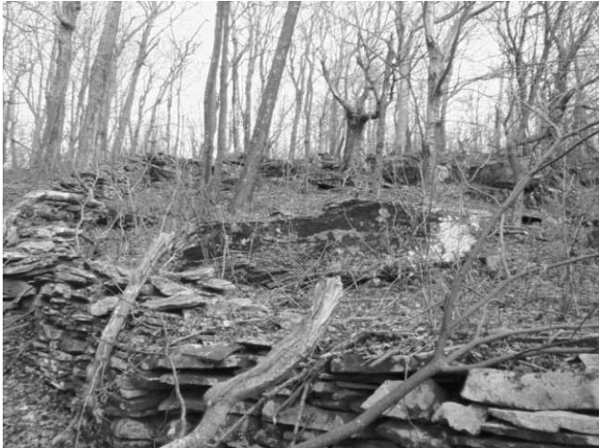
Looking up the wall enclosure from the north
